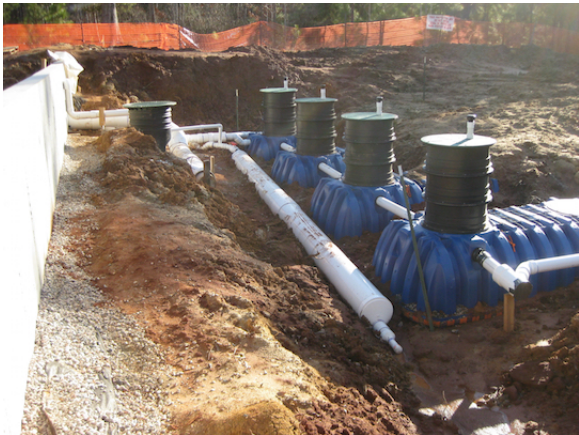
Infiltrator IM-Series Potable Water Tanks in a rainwater capture and reuse system
