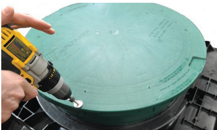
Fasten the lid to the riser with screws provided prior to backfilling.
