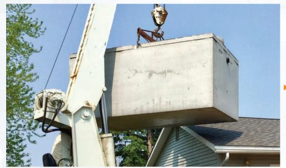
Concrete tanks require heavy equipment to transport and haul.
