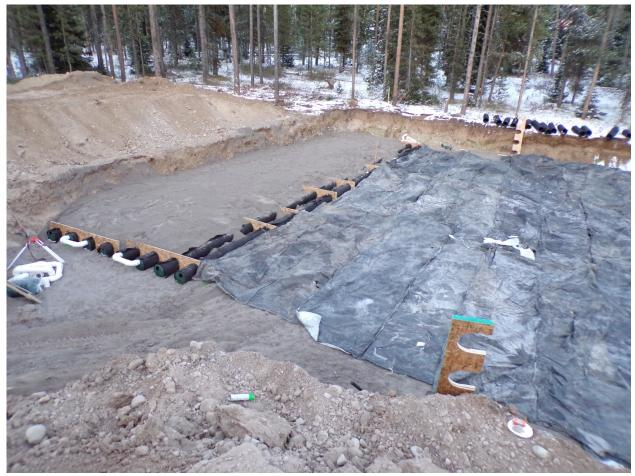
AMK Ranch selected a 6,500-gallon per day combined treatment and dispersal advanced enviro-septic (AES) treatment system with 3,120 linear feet of AES pipe.
