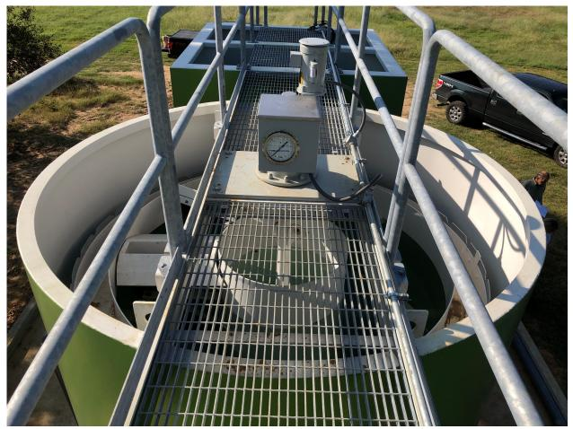
The Jellystone Park package plant processes wastewater via an extended aeration and oxidation process that purifies the sewage using naturally-occurring bacteria to destroy the organic compounds.
