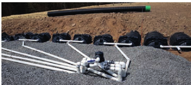
In the Forest Lakes installation, the effluent is time-dosed on an intermittent basis using pressurized micro-dosing, to a multi-celled, soil dispersal system that incorporates Infiltrator Quick4 Plus Standard Chamber laterals in an area bed arrangement. Photo by Infiltrator
