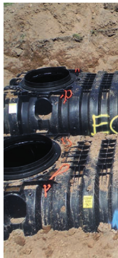
Right: The IM tanks with the ECOPOD-N treatment system were installed behind the house by lifting into place with a mini-excavator. The use of low-profile chambers in the drainfield eliminated the need for imported capping fill. Installation and final grade resulted in negligible impact on the existing lawn.
