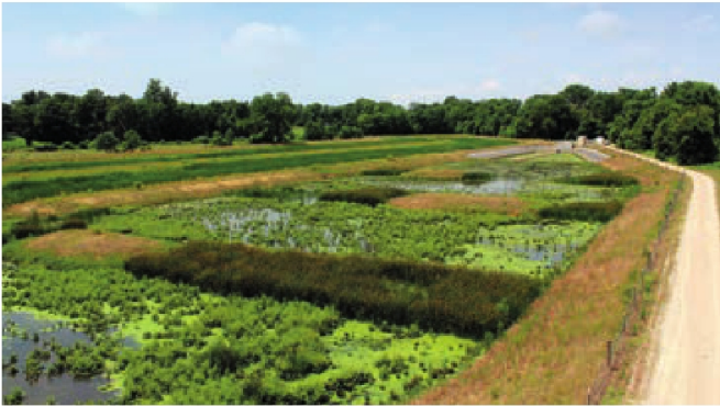
The future engineered wetland site is seeded with specific species of vegetation that will thrive in the wetland environment and allow evapotranspiration and nutrient uptake. Photo by Infiltrator Water Technologies
