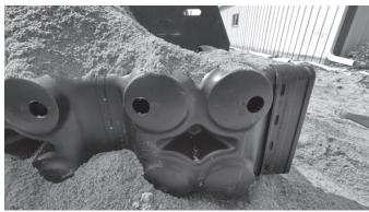
**5.** Start to backfill the system from the edges first. Keep sand away from the open ends of the system. Once system sand is holding system in place proceed to step 6.
