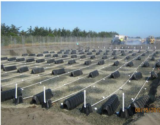
A new treatment plant and chamber drainfield system designed by Aaron Speakman of The Dyer Partnership Engineers was approved and constructed to treat, convey, and discharge the final effluent meeting Clean Water Act regulations, the WPCF permit, and the limits set forth in the NPDES permit.
