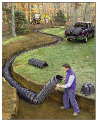
Infiltrator chambers are the original plastic leachfield drainage chambers.
