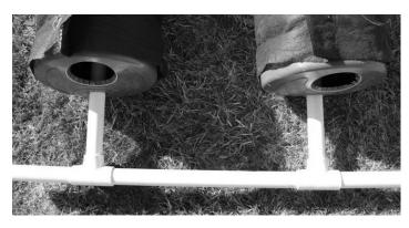
9. Install the 4" manifold for venting and make sure you are properly backfilled with system sand.
