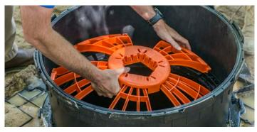
**Note:** If the Safety Star is installed at the riser-to-tank connection, the five screws used to fasten the risers to the tank also secure the Safety Star. The Safety Star is designed to allow up to a 4" (100 mm) pumping hose to enter the tank while installed, allowing for ease of maintenance without removal.
