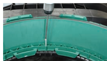
Screws required for riser to tank connection only.
