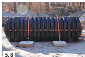
Position straps on tank.
