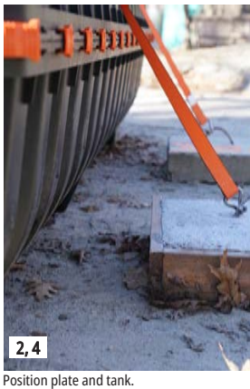
Position plate and tank.
