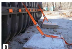
Connect strap to plate.
