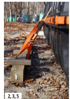
Position beam and tank.
