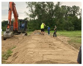
The installation provided an opportunity for the contractor and area health officials to learn about the AES product and how it is installed. The system blends in naturally with the site grading, eliminating the large hump associated with traditional mound systems and provided ample room on site for the owner's
