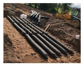
A 900 square foot Infiltrator ATL C-33 system was installed at a six-inch depth. Due to the requirement to have two feet of workable soil before groundwater, the four-inch size of the ATL and the taller invert were ideal. The passive ATL system eliminated the need for a pump system and operates even if the power is interrupted. The installer boxed out the bed system, installed 300 linear feet of Infiltrator ATL, and backfilled the system in one day.
