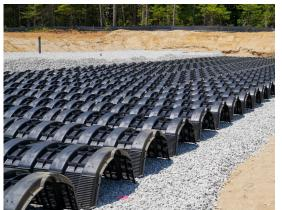
Other system designs and drainfield chambers were considered, however the Infiltrator High Capacity H-20 chamber, which is rated for 32,000 lbs. per axle, was selected to accommodate for potential vehicle traffic over the system including larger vehicles if needed. The subsurface discharge allows the future use of the land as open space to be enjoyed by all, there will be a preserve with several foot trails. Operation and maintenance will be minimal for the disposal beds.
