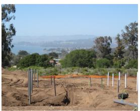
The disposal and recharge system utilizes approximately 20,000 linear feet of Infiltrator chambers installed in a series of trenches that offer enhanced infiltrative surface area to return the treated effluent back into the soil to replenish groundwater supplies.
