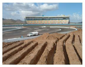
posed some space restrictions and made for an oddly shaped area for the leachfield. The chambers offered more design flexibility when compared to the proposed stone and pipe systeme and were faster and easier to install.
