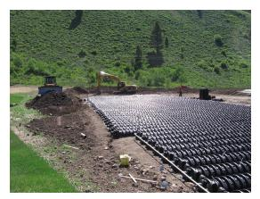
main. Effluent is then conveyed to a separate pump chamber and the pressurized network. Isolation valves within the network were incorporated to facilitate system operation and maintenance and to minimize service interruption.effluent will enter the bed and filter through the soil then into the groundwater.
