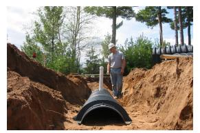
to a distribution box to provide proper distribution to the drainfield. Each individual system pumps the effluent to its own drainfield. Combined, the two drainfields include 658 Quick4 Standard chambers. Observation ports at surface level have green poly covers so they are not visible, nor do they interfere with the recreational use of the area.
