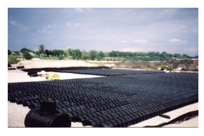
A concern from the start was the fluctuating ground water levels in the area, which could result in the bed becoming submerged. The system was designed so that the hydraulics of the plant ensures that the plant effluent will enter the bed and filter through the soil then into the groundwater.
