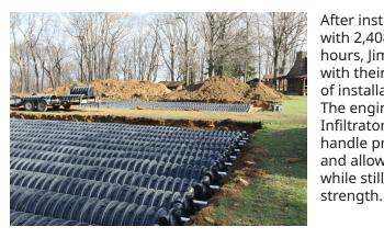
After installing 580 Infiltrator chambers in two beds, with 2,408 LF of SCH40 PVC pipe in less than six hours, Jim Mack Excavating was impressed with their ease of installation, speed of installation, and transportability. The engineer was pleased with Infiltrator chambers ability to handle pressure distribution and allow air movement, while still having
