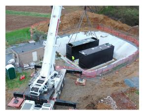
The system design utilized a Bardenpho process with flow equalization, a pre-anoxic tank, aeration tank, post-anoxic tank, polishing tank, dual-hopper bottom style clarifiers, a solids holding tank and disinfection. The treated effluent discharges directly into the Conestoga River adjacent to the property. Although not required by the permit, the system treats to aggressive total nitrogen and total phosphorous goals.
