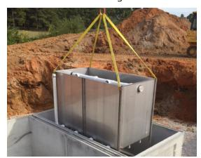
primary tanks. A spray disposal system was also supplied by Infiltrator, complete with effluent pumps, spray heads, tubing, controls, and all necessary valves and fittings. Concrete tanks supplied by a local precaster.
