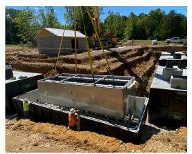
or subsurface land application system, or construction of a package wastewater treatment plant. The system needed to be designed for an average daily flow of 20,000 GPD with peak flows of up to 25,000 GPD. A 20,000 GPD ECOPOD Advanced Wastewater Treatment System with Geoflow dip irrigation was selected for the final design.
