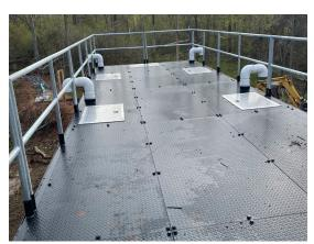
An ECOPOD Advanced Wastewater Treatment System was designed to meet the new ammonia effluent requirements of 1.25 mg/L (summer) / 2.75 mg/L (winter). A single-compartment tank with an ECOPOD E3400D was installed in an epoxy coated steel tank.
