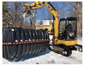
To prevent the soil from freezing prior to the early March 2018 installation, in fall 2017 the site was covered with frost blankets. The installation went smoothly with daily clearing of all piles of dirt to prevent overnight freezing presenting the hardest challenge.
