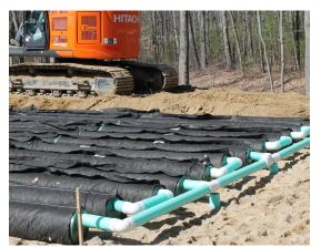
Presby Maze installed in one tank to increase efficiency by lengthening the flow path and further trap suspended solids. During ground preparation for the replacement system, three-feet of silty clay on top of the old system that was contributing to the perched water table was removed.
