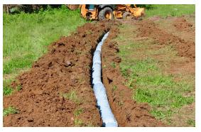
A pressurized system was required by the County because the system size was over 500 feet. The first of a possible three systems of equal size to be designed and installed at Camp Cedar, the wastewater treatment system serves the main house and two of the bunk houses at the camp. The system incorporates four zones controlled by a splitter valve for equal disribution.
