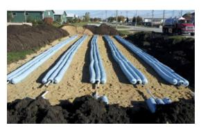
LPP dispersal field size is calculated at 5 square feet per linear foot of EZflow 803H LPP geosynthetic aggregate bundles.
