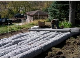
The additional fill removed during the tank installation was used up hill from the at-grade treatment area to blend the system into the yard. Once completed, other than the inspection ports, the system was constructed to disappear into the landscape.
