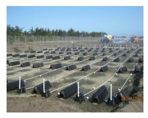
A new treatment plant and chamber drainfield system designed by Aaron Speakman of The Dyer Partnership Engineers was approved and constructed to treat, convey, and discharge the final effluent meeting Clean Water Act regulations, the WPCF permit, and the limits set forth in the NPDES permit.
