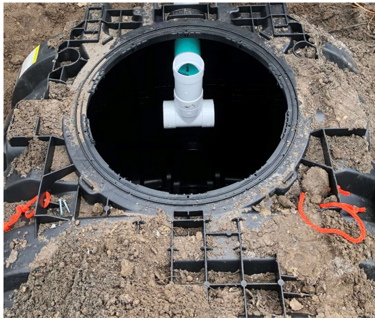
Figure 8: 4" Discharge Tee Assembly
