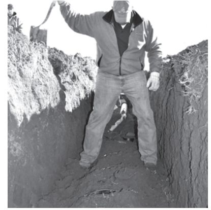
Walking in the fill along the trench edges
