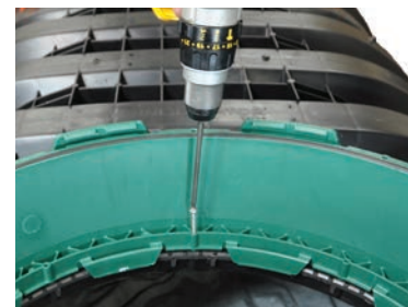
Screws recommended for riser to tank connection only.
