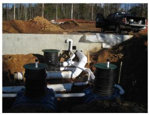
interconnected at their base on alternating ends to keep the freshest water moving thru to the last tank. The last tank has overflow pipes equal in size to the inlet pipes. Both overflows are fitted with an overflow siphon (p-trap) and rodent guard.
