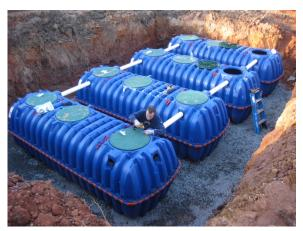
The system is designed with four, Infiltrator IM-1760C, 1787-gallon potable water tanks installed in series and connected at the bottom to function as one large tank and to yield a total storage volume of over 7,000 gallons. The Infiltrator tanks are NSF/ANSI Standard 61 (NSF 61) certified for potable water storage meeting a rigorous set of national standards to ensure potable water storage safety.
