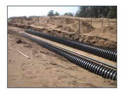
Final Disposal for the community of Los Osos includes a community drainfield that will provide much needed groundwater recharge to minimize saltwater intrusion.
