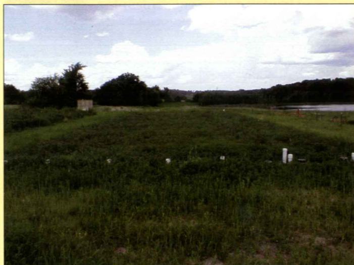
The wetland system at the Fields of St Croix after completion. Image: Infiltrator
