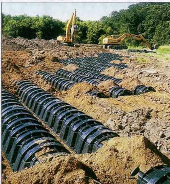
**A large chamber system provides final disposal and treatment for a constructed wetland treatment system.**
