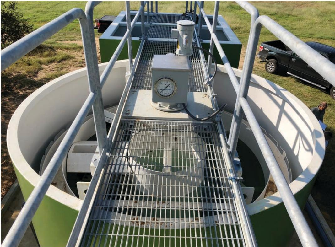
**The self-contained wastewater treatment unit, called a Delta Packaged Treatment Plant, (seen here at Yogi Bear's Jellystone Park in Texas) can be accessed from the top.** Infiltrator Water Technologies
