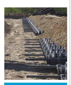
Sized for 1,353 cubic meters per day, the Omemee modular disposal system design includes the existing flow and allows for expansion for future growth.
