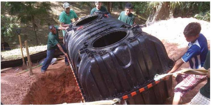
Plastic tanks are becoming more common in decentralized wastewater treatment systems. Ease of shipping and installation coupled with high strength, water tightness, and materials that are inert to septic gases have helped the industry. In this rural system, the Infiltrator IM-Series plastic tank is lowered by hand into place at the installation location. Photo by Infiltrator Systems
