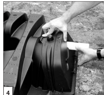
Place end cap over inlet end.
