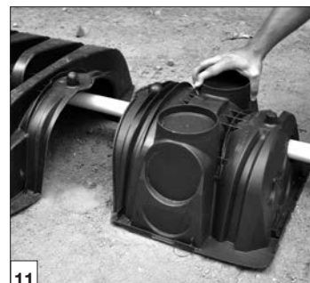
Lateral pipe through end cap.
