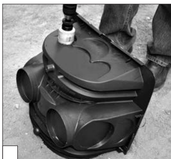
Drill pressure pipe hole.
